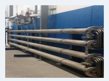
The heat reclaimer, installed by Kemco Systems of Clearwater FL, preheats incoming water by passive transference of heat to within 5 to 10 degrees of the wastewater stream. This reduces the energy required to actively heat water and substantially reduces the temperature of the outgoing wastewater. Not only does this heat recovery system benefit the local water systems and the balance of aquatic life, but the anticipated reduction in greenhouse gas from energy production is 1,892 MTC02e annually.
